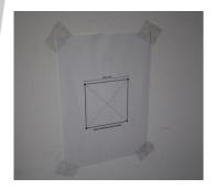
1) Mount provided VESA template to surface and in ideal location. This is often behind and above screen walling mounting brackets, in order that the player is hidden from sight once the screen is in place
